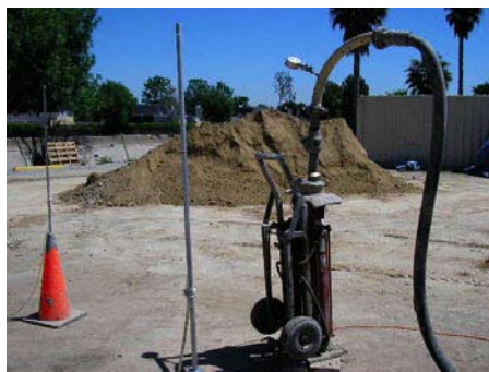
The grout injection equipment with manometers for level survey.
