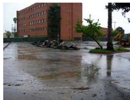
The site was covered with asphalt before beginning the grouting process.
