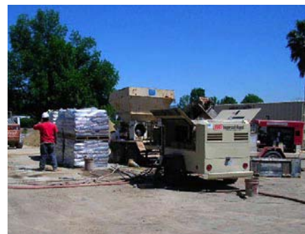
Onsite portable batch plant used with the generator to mix grout.
